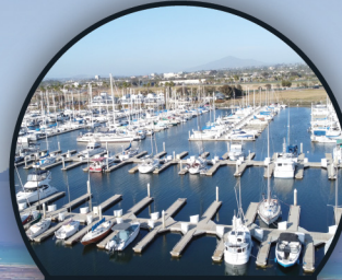
MARINA SAFE HARBOR SOUTH BAY
