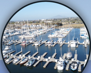
MARINA SAFE HARBOR SOUTH BAY
