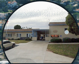
ROSEBANK ELEMENTARY SCHOOL
